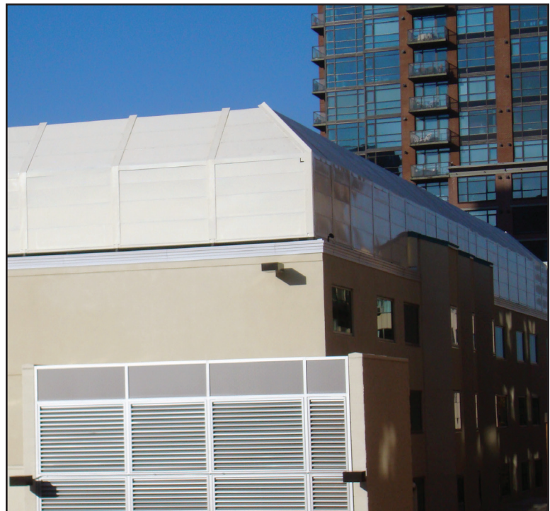
Roof Top Equipment Barrier
