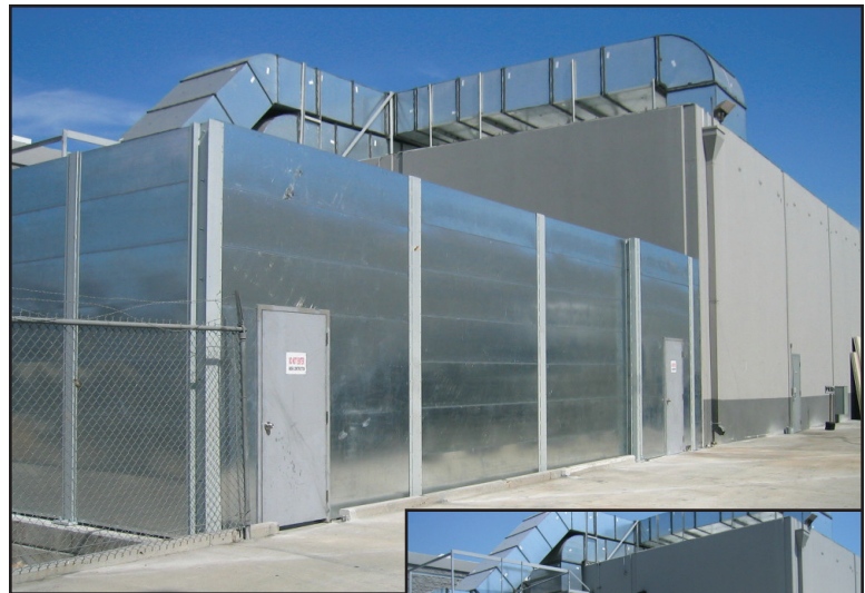
Chiller Barrier Wall System, Before (right), After (above)
