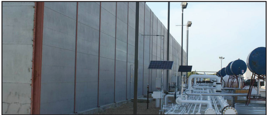
NOISEBLOCK™ Barrier Wall Midstream Compressor Station
