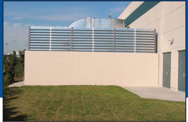
Equipment Yard Barrier Wall
