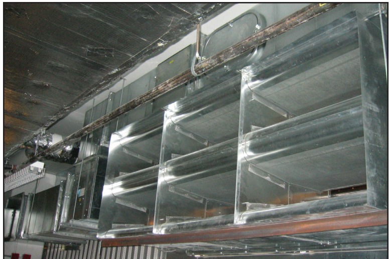
Rectangular Duct Silencers - KCRS-F/3
