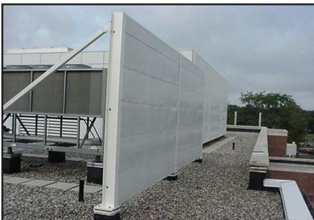
Roof Top Barrier Wall
